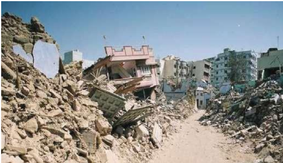
Housing Damage after the 2001 Gujarat Earthquake
